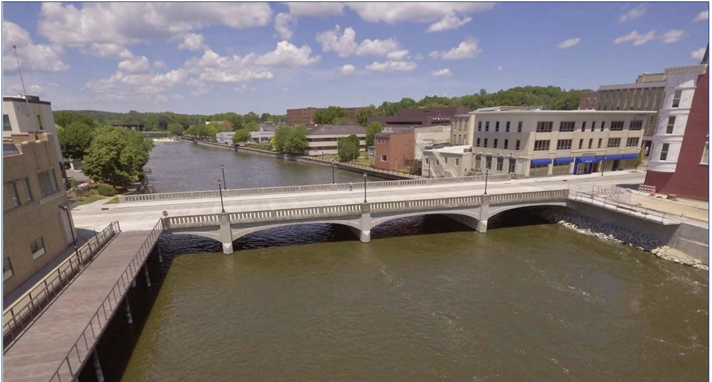
Completed bridge over the Rock River, Janesville.
