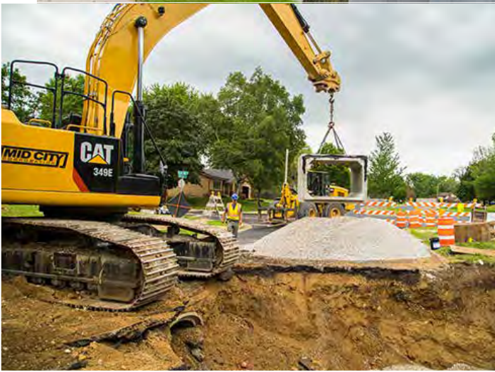
Ready-to-install box culvert sections saved valuable time and reduced road closures.
