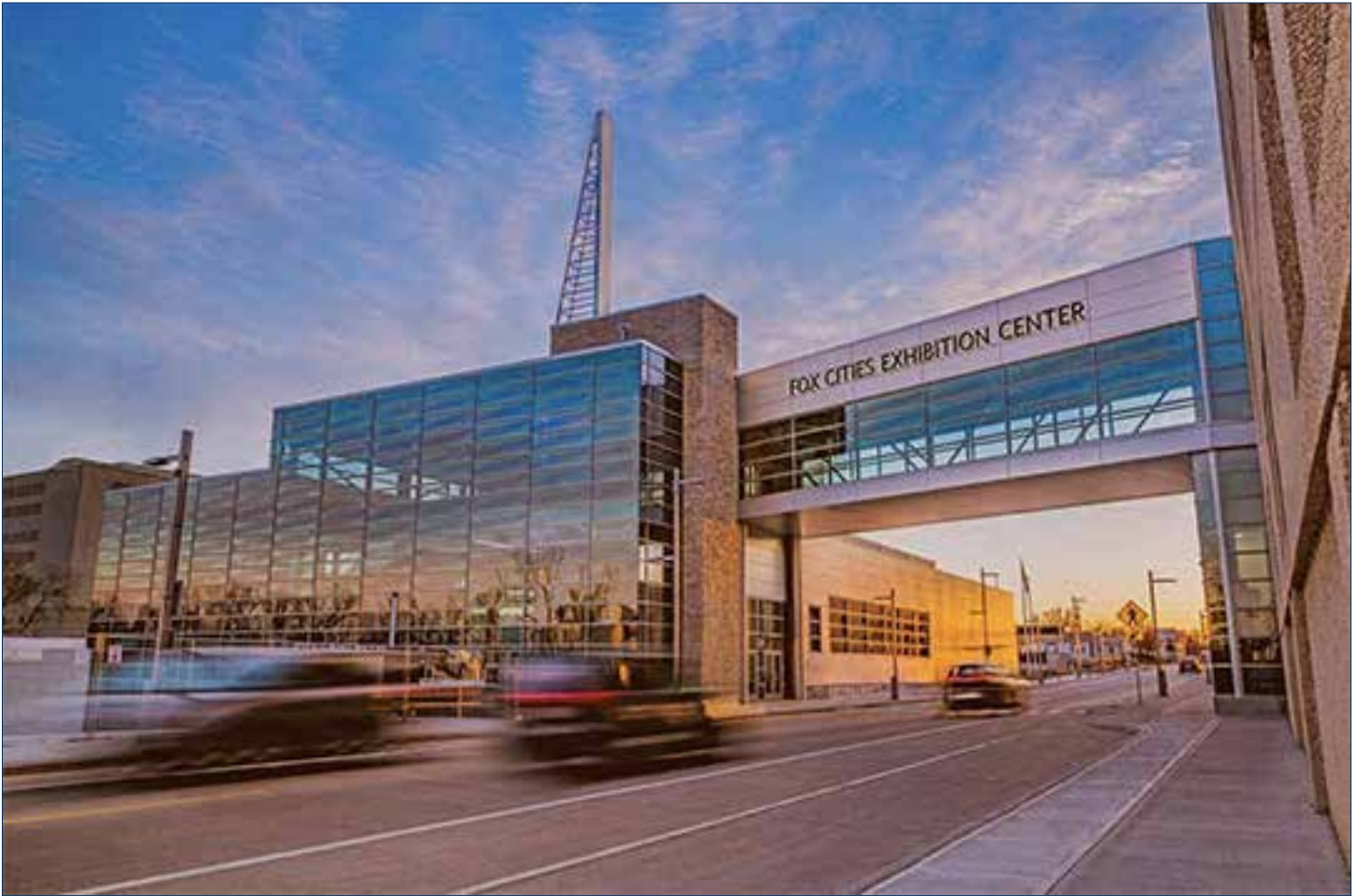
The Fox Cities Exhibition Center in Appleton is headquarters for the 2022 Spring Conference.
