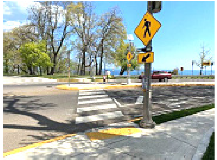
“Danish Offset” crosswalks provide better sight lines for pedestrians to observe oncoming vehicles.
