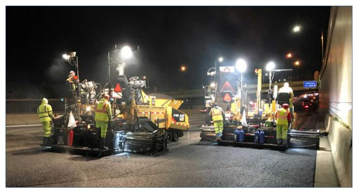
*Reduced traffic volumes and full system lane closures allowed for an increased workforce to double the number of peak production hours each night, completely eliminating the need for unnecessary transverse cold joints.*
